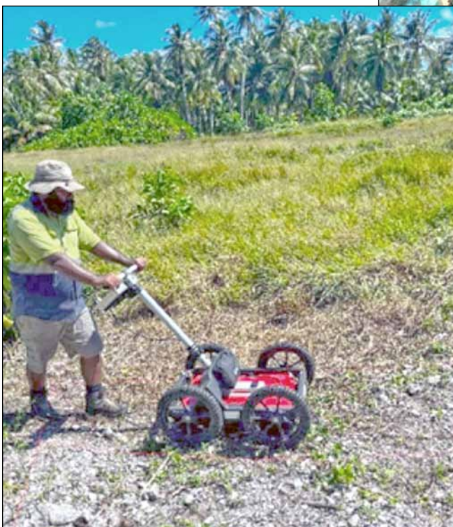
SPC's Senior Hydrogeologist, Amini Loco, is screening the soil using UXO machine to detect possible mines across the proposed construction site adjacent to the runway.
