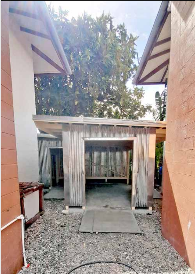
North Delap School drinking water station building.
