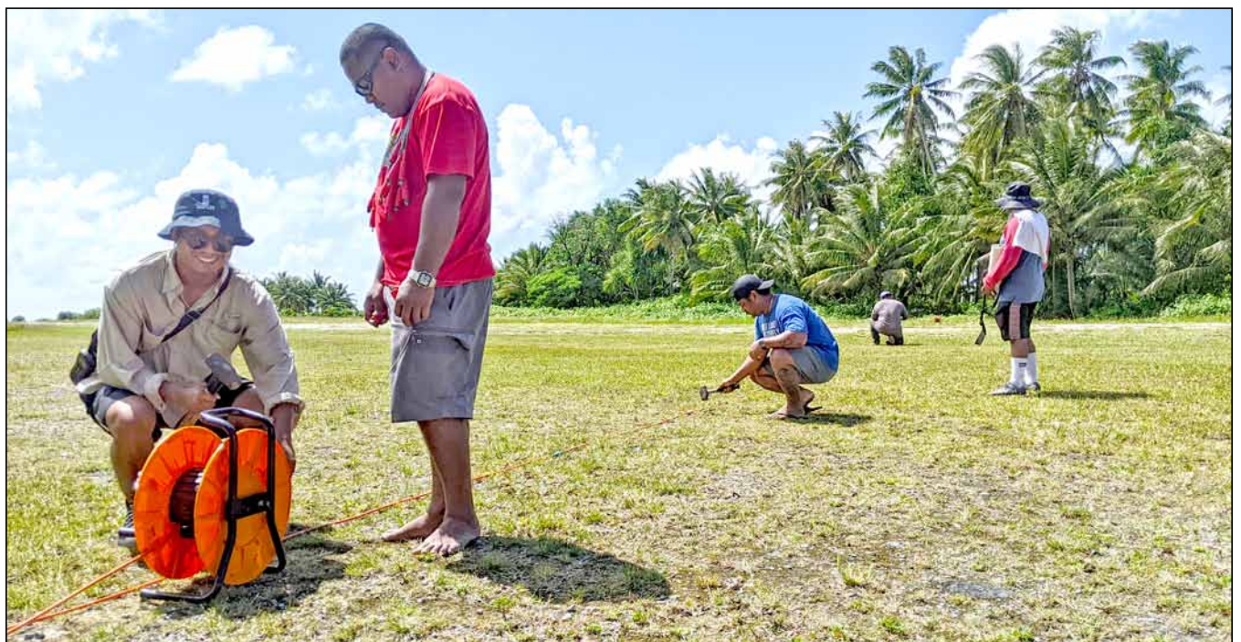
The team laying out the electrical resistivity cables and hammering in electrode rods across Woja airport runway.
