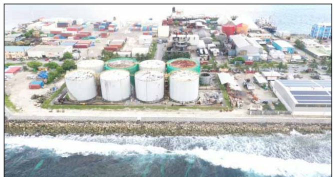
MEC Armor Rock and Seawall upgrade.
